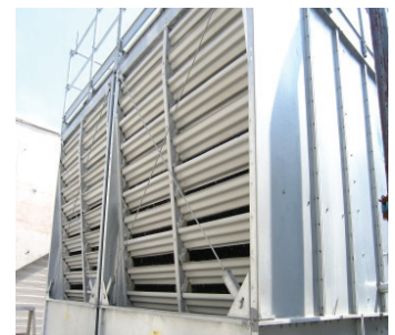
Drained Cooling System
