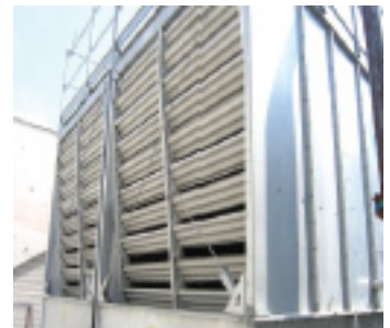
Drained Cooling System
