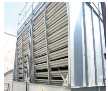
Drained Cooling System
